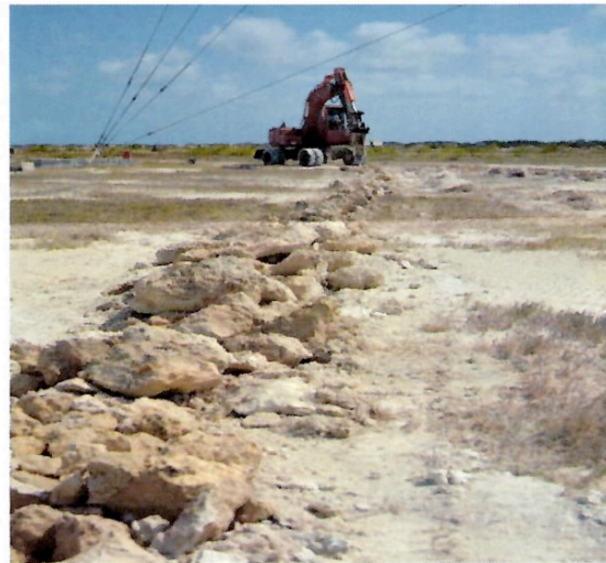
Trenching for feed lines
