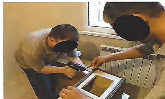
Central Asia co-workers as we prepare ventilation for new studios.
